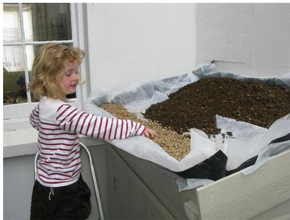
Another layer of fleece, and you can put the substrate in. BUT FIRST, put a deep layer of vermiculite (blown clay) at the front to help with drainage.
