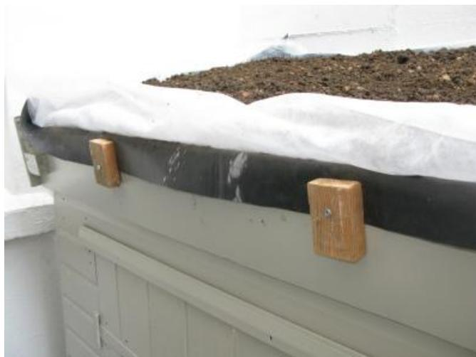
Fold over the excess liner at the front, and fix behind the spacers you screwed on earlier. This is the lip that excess water will drain over.
