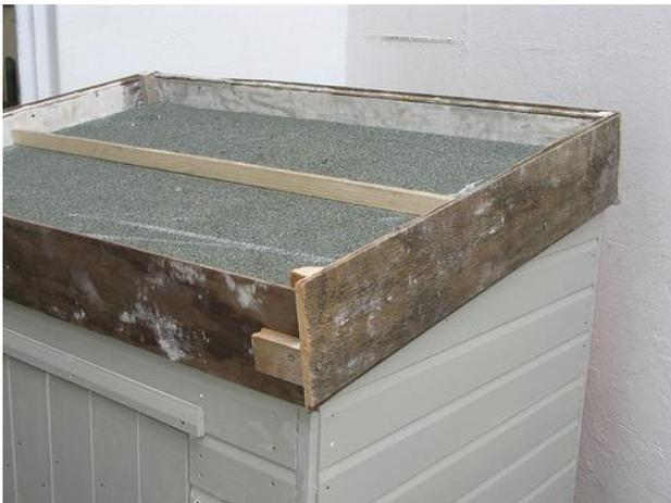
The batten (pale cross-piece) helps stop the substrate slipping down the sloping roof. Nail or screw it to the side boards.
