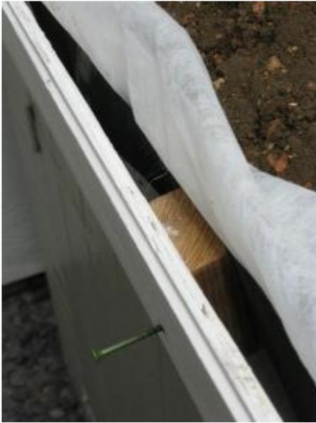
Screw your finishing fascia onto the spacers, using board the same width as the side and back pieces.
