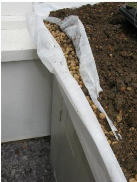
Get the cut off strip of fleece, and put over the vermiculite. Push substrate on top.
