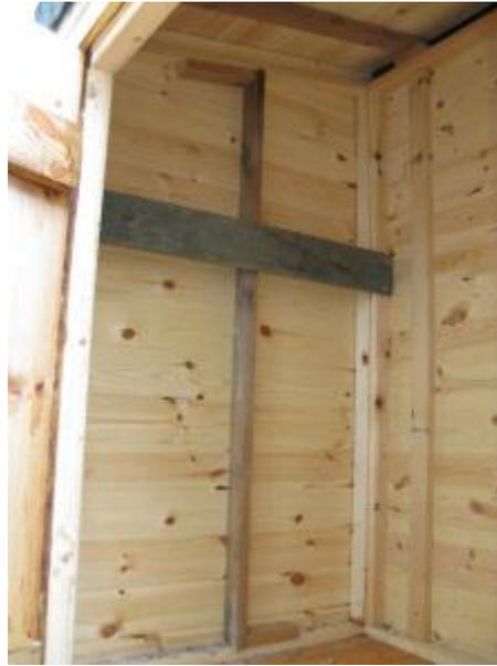
Use battens (here shown as the darker coloured cross-pieces on the sides) to strengthen the shed. This is to enable it to take the extra weight of the roof and stop it twisting.
