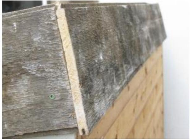
Showing the back board fixed. It is screwed to the roof joists, and the short upright pieces joined to the side boards.
