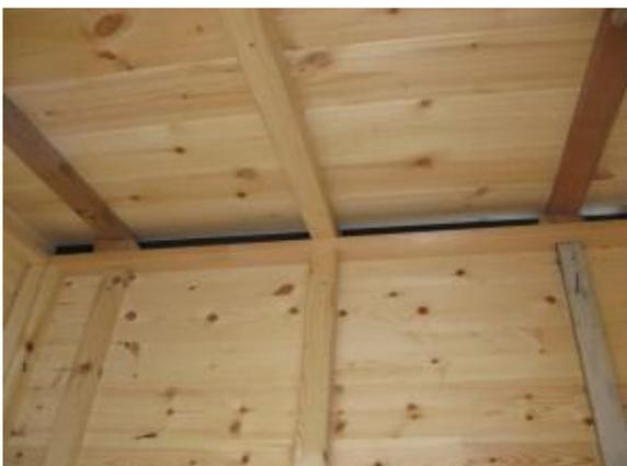
Extra joists screwed in to support the weight of the substrate on the roof deck.
