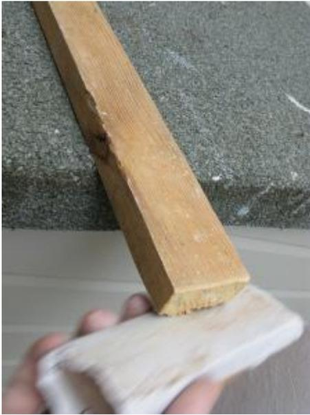
Make sure you sand all timbers used for the roof to minimise the risk of splinters causing leaks.
