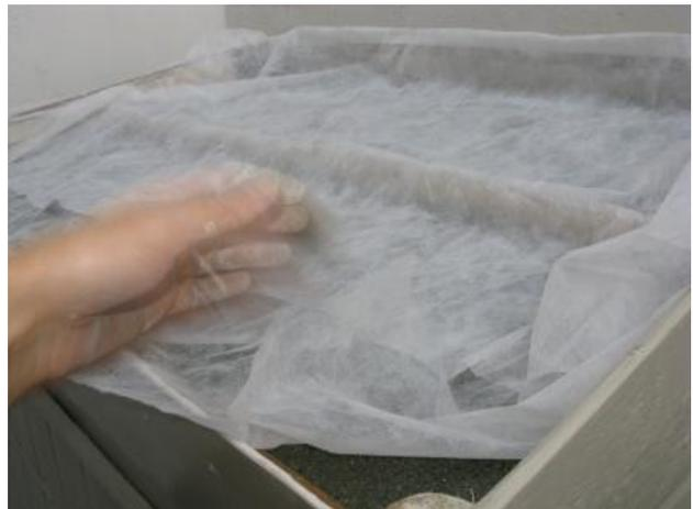
A layer of fleece helps guarantee against sharp edges puncturing the liner.
