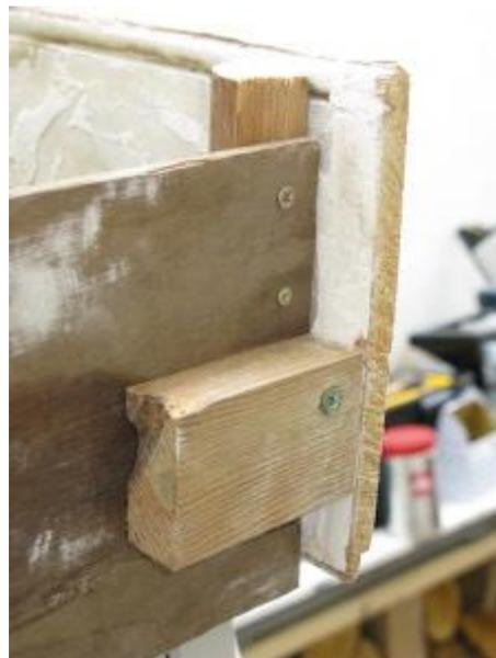
In this design, excess water will run over a hidden fascia, behind the main fascia board. Spacers are used to separate the two facias. Use three or four spacers like this.
