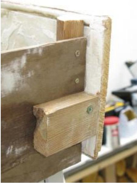
These boards (white in this picture) make up the sides and back of the green roof. I used old skirting boards - slightly thicker boards would have been stronger, but heavier. They determine the depth of substrate you will have.
